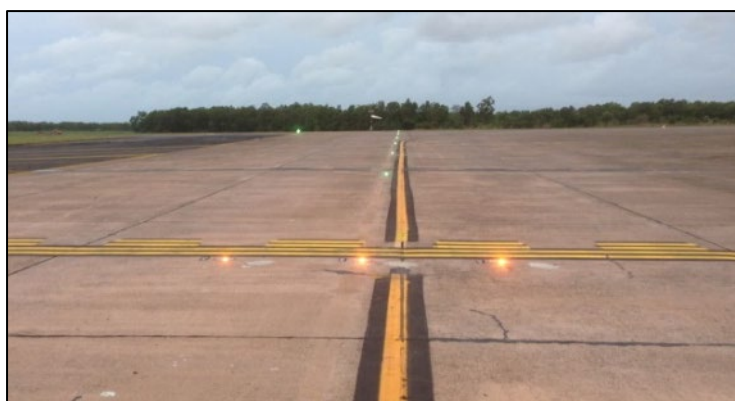
RWY Holding Position Lights
