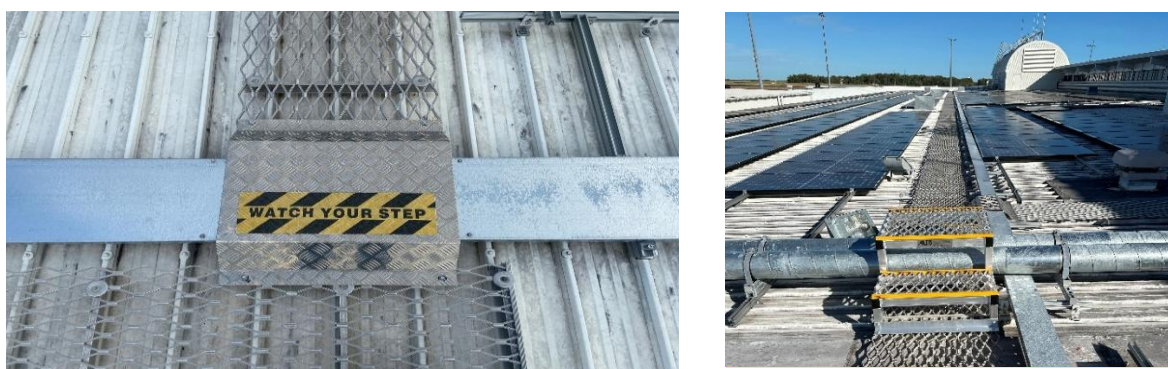
Photo 4.3 – Trip hazards (Step over) – highlighted or marked with strip
