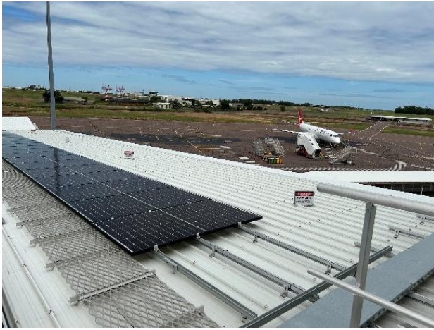
Photo 4.6 – Unprotected edges – No access outside designated walkways without a Working at Height Permit approved by the ADG Safety team.
