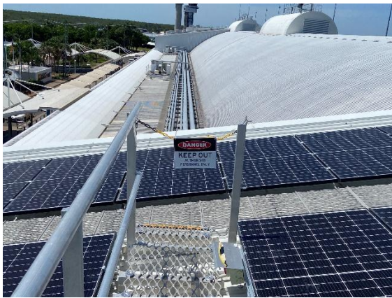
Photo 6.12 – Area B West – Prohibited access to eastern sloping walkway from bottom walkway– Must have a Working at Height Permit approved by ADG Health & Safety Manager or approved delegate.
