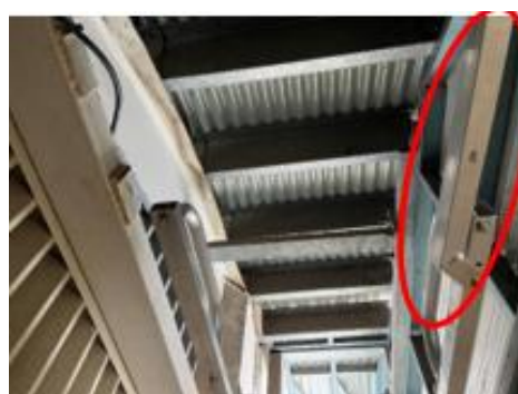
Photo 6.32 – Area Central PR filter – Guard rail open position
