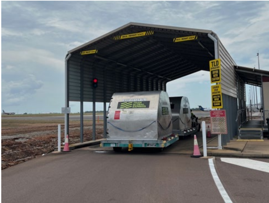
Eastern ACP Inspection
