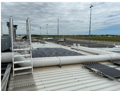
Photo 6.4 – Area A – highlighting east roof live edge
