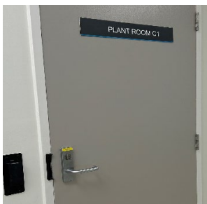
Photo 5.2 – Plant Room 1 st floor
