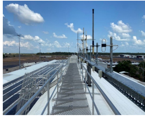
Photo 6.28 – Area PR – Radiation Hazards
