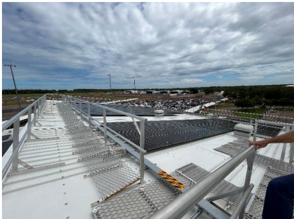
Photo 6.8 – Area B West – Roof walkways Western end
