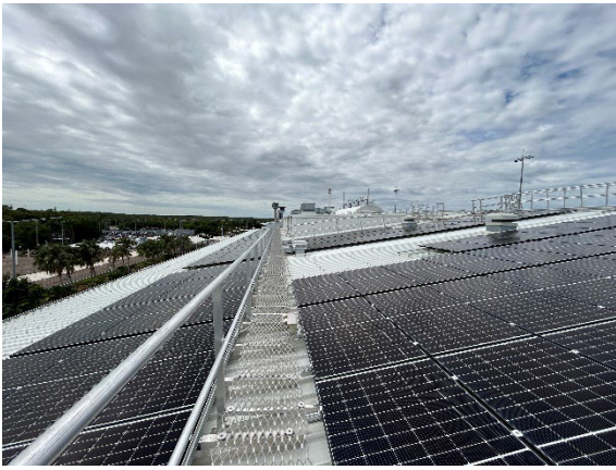
Photo 6.10 – Area B West – View from walkway facing East
