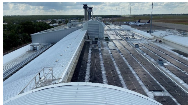
Photo 6.23 – Area E – View from Area PR Central facing East
