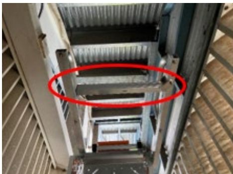
Photo 6.31 – Area Central PR filter – Guard rail closed
