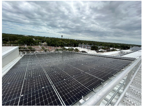
Photo 6.11 – Area B West – View from walkway facing North
