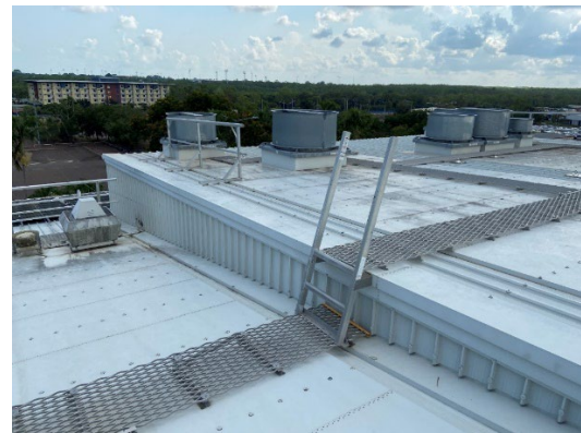
Photo 6.21 – Area D East – Step access Area B to Area D East
