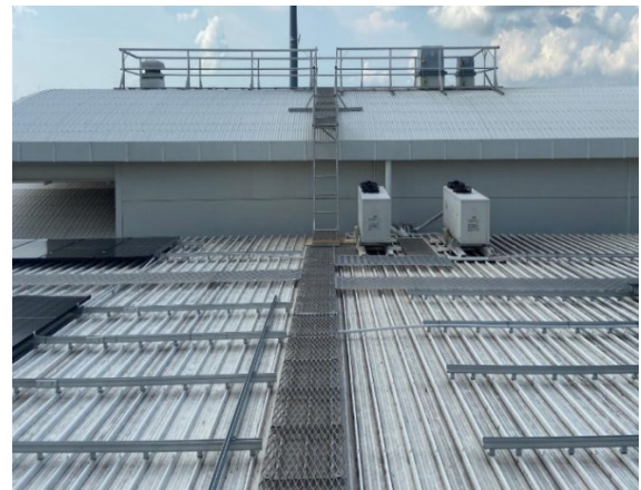
Photo 6.25 – Area F – Ladder view from Area A to Area
