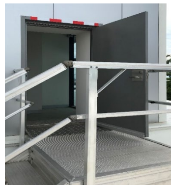
Photo 5.5 – Access door to roof
