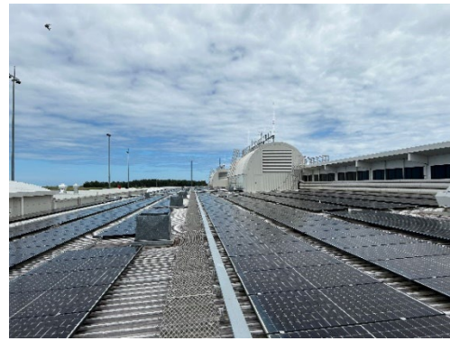
Photo 6.3 – Area A – looking west
