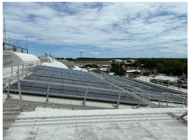
Photo 6.15 – Area B East – Western view from top roof
