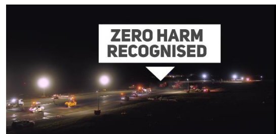
Alice Springs Airport runway resurfacing project
