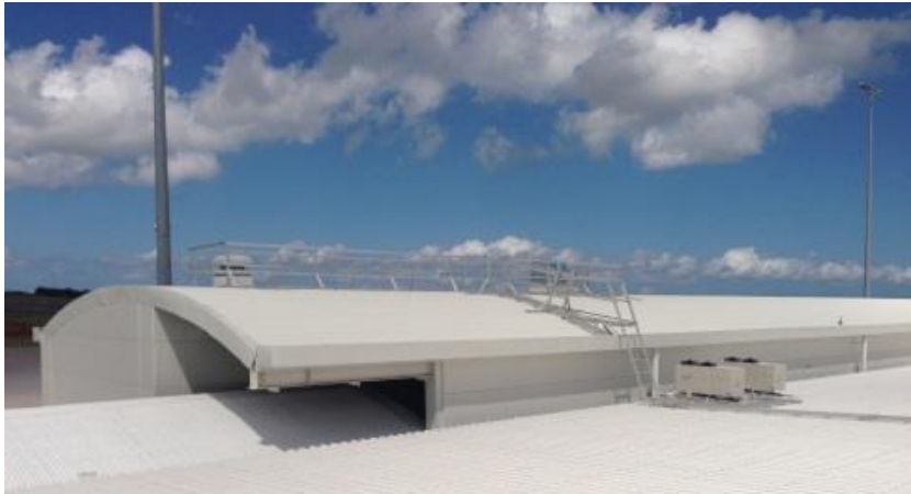
Photo 7.4.6 - Area F access
