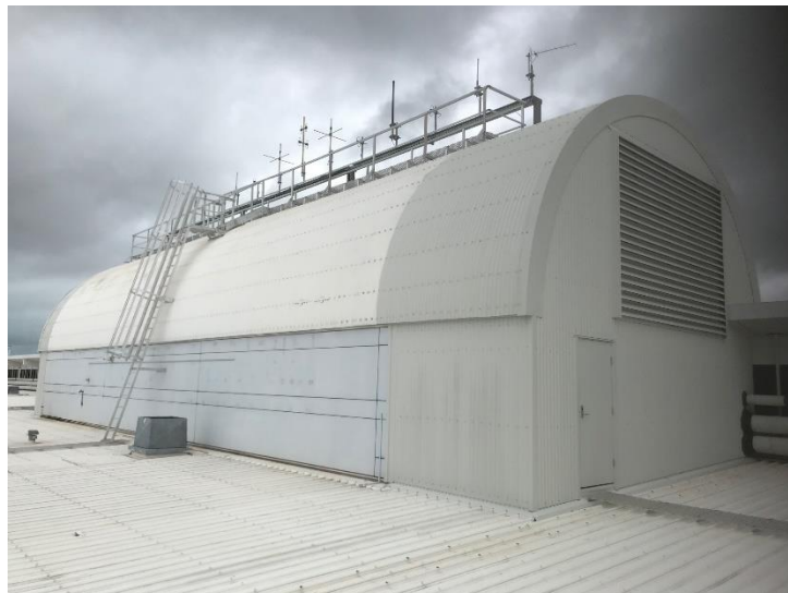
Photo 7.4.7 – Area PR – Plant Room Roof access
