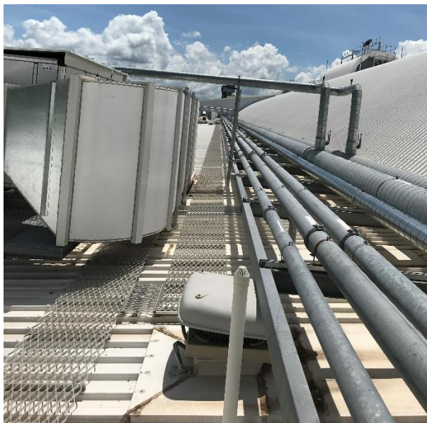
Photo 7.4.3 – Flat roof landside
