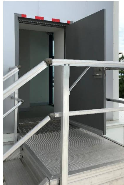
Photo 7.4.9 (ii) – Access door to roof
