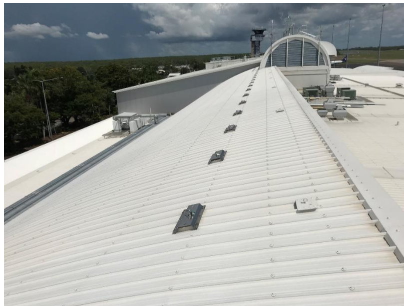
Photo 7.4.5 – Area E roof
