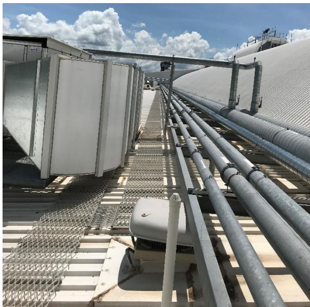
Photo 7.4.3 – Flat roof landside
