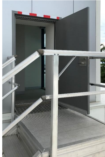
Photo 7.4.9 (ii) – Access door to roof
