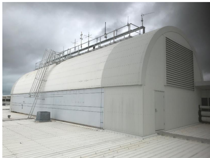
Photo 7.4.7 – Area PR – Plant Room Roof access
