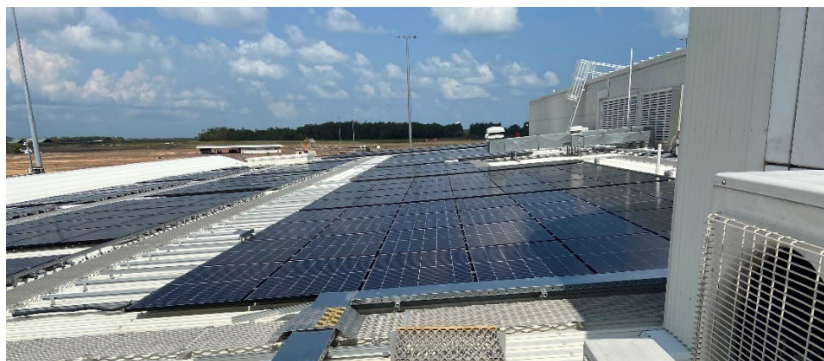
Photo 4.4 – Burn hazard – When working near solar panels workers must wear gloves
