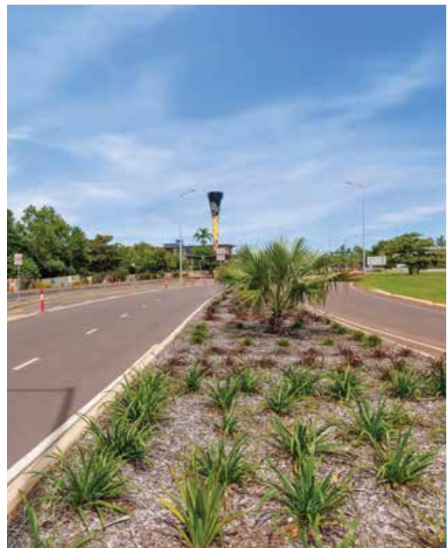
Smart irrigation installed to landscaped median strips during road network upgrades
